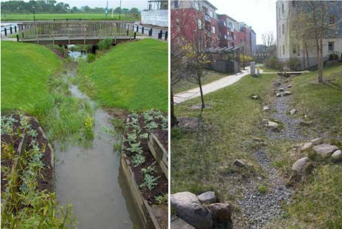
48. We will welcome developments integrating sustainable urban drainage which is designed to be an attractive and interesting feature of the environment.
